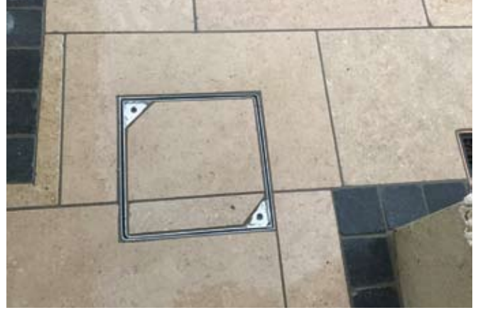
Recessed Manhole Cover Used Within a Landscape Project
